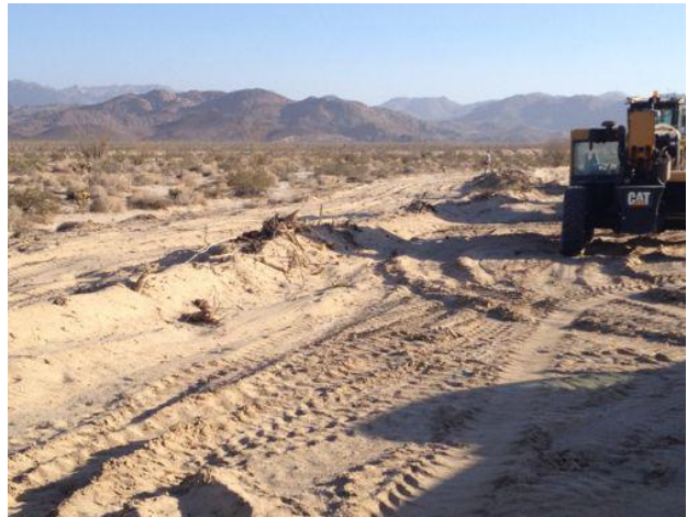
Photo 3: Topsoil being salvaged onsite in accordance with MM Veg-2b.
