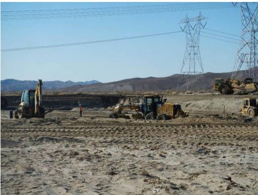
Photo 7: Heavy equipment is utilized to establish the 30-acre substation/switchyard pad site.
