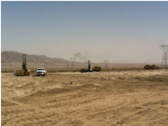
Photo 3: Drill rigs completing geotechnical testing activities at the 30-acre substation/switchyard.
