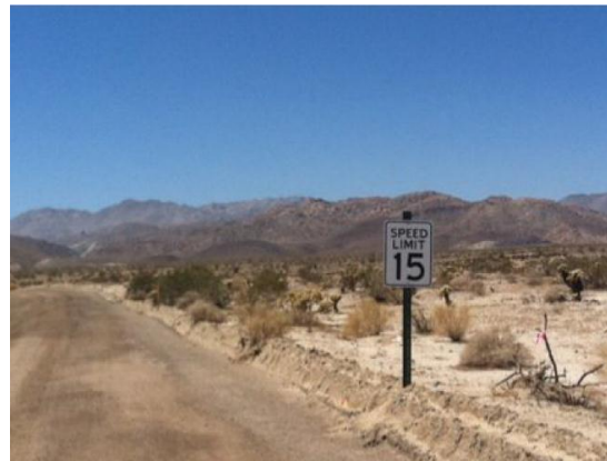
Photo 4: Signage is placed along the access road between the temporary laydown yard and the substation/switchyard to inform construction crews vehicle speeds are limited to 15 miles per hour.
