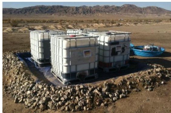
Photo 8: Secondary containment is utilized for storage of hazardous materials onsite during construction.
