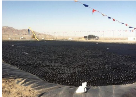
Photo 6: Armor balls have been placed along the water surface at the temporary water pond in accordance with Section 4.2 of the Raven Control Plan (MM-Wild-1j).
