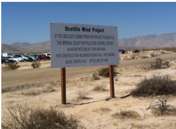
Photo 3: Public informational signage has been placed along S-2 and Dos Cabezas Road to provide the public with contact information during construction.
