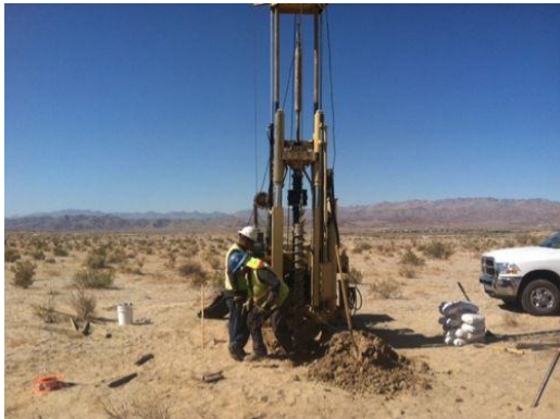
Photo 7: A drill rig completing geotechnical activities within the approved work limits.
