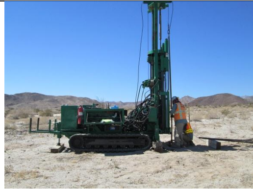
Photo 8: A drill rig completing geotechnical activities within the approved work limits.
