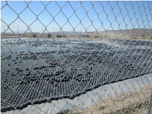
Photo 7: Armor balls have been placed on the surface of the temporary water pond in accordance with the Raven Control Plan (MM-Wild-1j).
