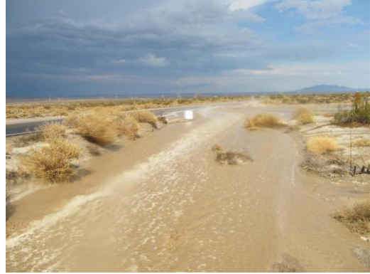
Photo 10: The rain event that occurred on 7.13.12 resulted in localized flooding as seen here at the intersection of County Route S2 and Dos Cabezas Road.
