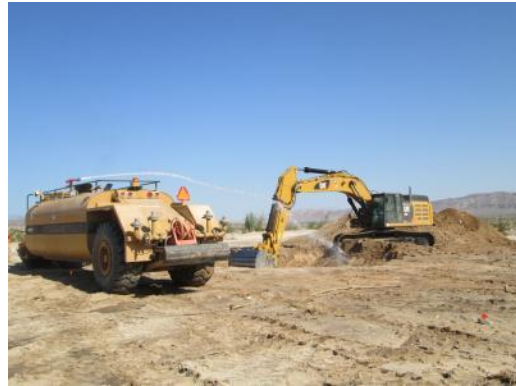
Photo 2: A water truck applies water during grading activities to minimize dust emissions in accordance with the Dust Control Plan.
