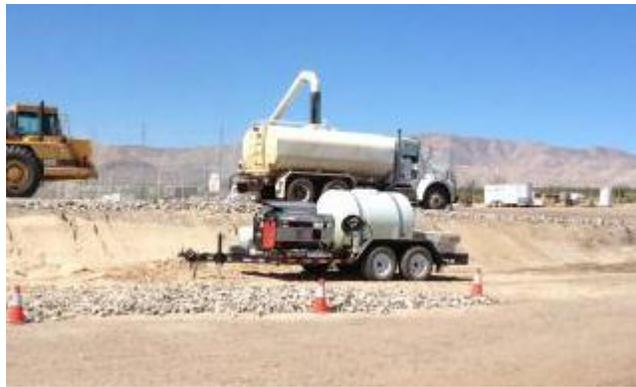
**Photo 3:** In accordance with the Integrated Weed Management Plan (MM-Veg-1d), a wheel wash station is located onsite to ensure vehicles and/or equipment that leave the site and are used on other sites are washed when leaving the site and prior to re-entering the site.
