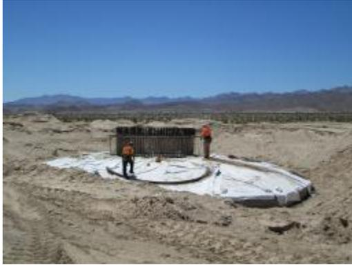
**Photo 5:** A crew completes construction activities at a wind turbine foundation.
