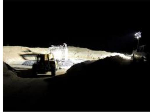
**Photo 6:** Crews complete nighttime work at wind turbine foundations. Lighting is pointed downward in accordance with the construction lighting mitigation plan (MM-VR-2).
