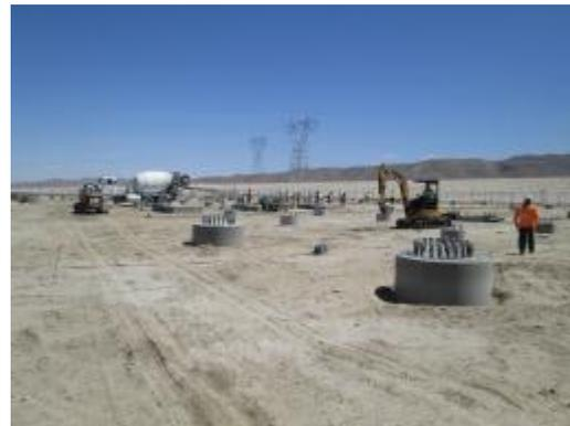
**Photo 8:** Construction crews complete foundations at the onsite substation that will be utilized for construction of substation components.
