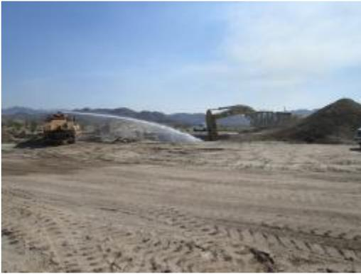
**Photo 1:** A water truck is utilized during excavation activities to minimize dust emissions.
