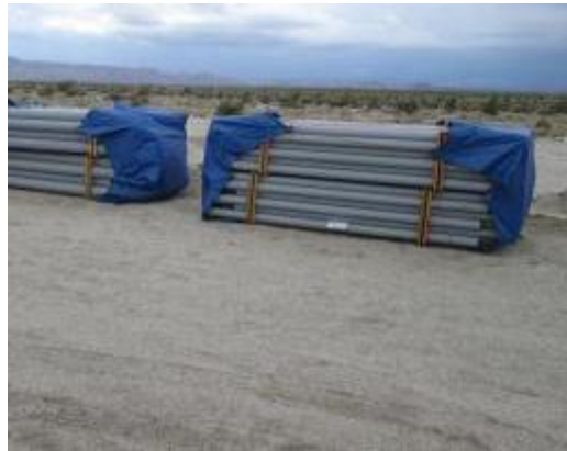
Photo 4: In accordance with MM-Wild-1m, construction piping is covered at the substation.
