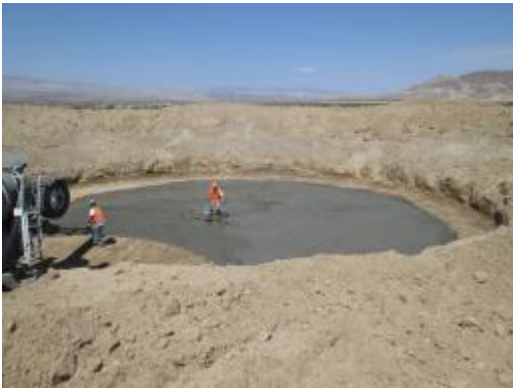
Photo 7: A base pour is completed at a wind turbine foundation.
