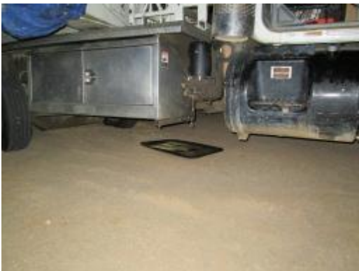
Photo 3: Drip pans are placed beneath construction equipment to minimize the potential for oils to stain soils along the ROW.
