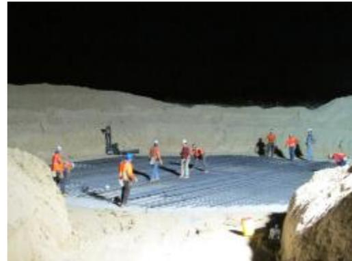
**Photo 8:** A crew completes a bottom mat at a wind turbine foundation during the evening hours.
