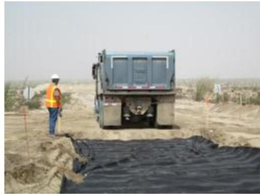
**Photo 2:** Stabilized construction entrances are established at the entryway to each wind turbine string from paved roadways. Stabilized construction entrances include a rock apron that reduces potential trac-out along paved roadways.
