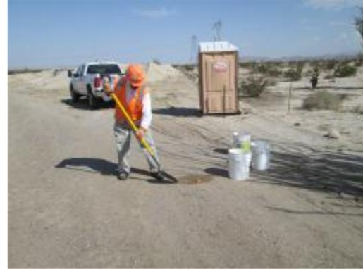
**Photo 6:** Crews remove stained soil along the ROW in accordance with the SWPPP (MM-Water-9).
