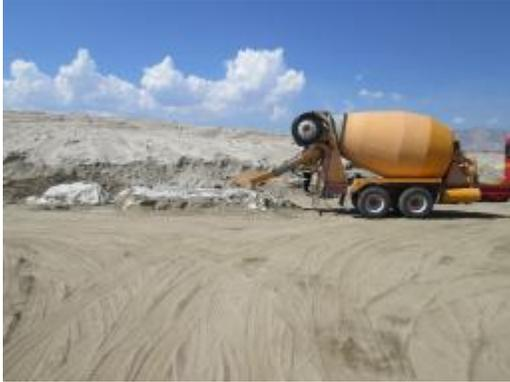
**Photo 5:** A concrete washout is utilized by cement truck operators to wash-out cement trucks along the ROW.
