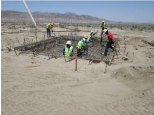
**Photo 7:** Foundations being constructed to support components for the Operation & Maintenance facility.
