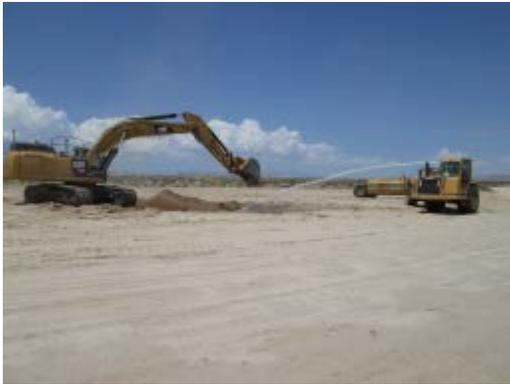
**Photo 3:** Water trucks are utilized during excavation activities to minimize dust emissions in accordance with the Dust Control Plan (MM-Air-1).
