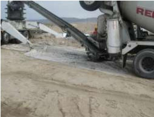
**Photo 3:** Plastic sheets are placed beneath concrete trucks and a conveyor belt to minimize the potential for concrete waste to be spilled onto the ROW during a wind turbine foundation pour.
