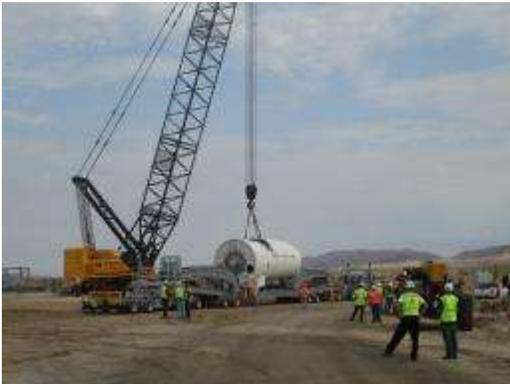
**Photo 7:** A crane is utilized to unload a nacelle from a haul truck to be staged along the ROW.
