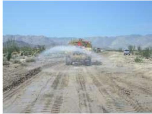
**Photo 2:** Water trucks are utilized during access road grading to minimize dust emissions in accordance with the Dust Control Plan (MM-Air-1).
