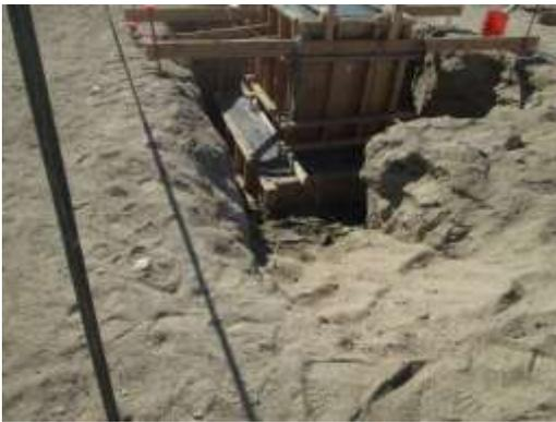
**Photo 3:** Wildlife escape ramps are put in place when excavating building foundations at the O&M facility in accordance with MM-Wild-1b.
