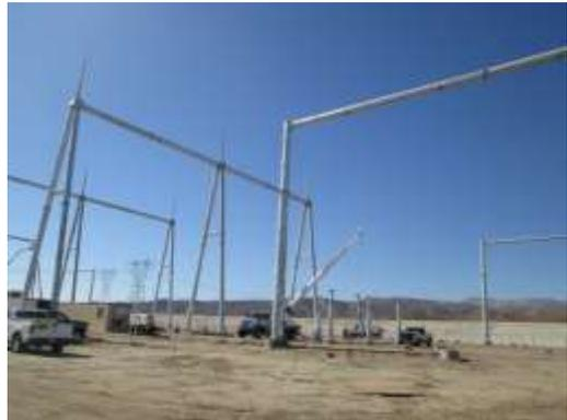
**Photo 8:** A frame structures are erected with cranes at 30-acre Substation/Switchyard.
