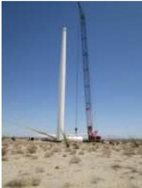
**Photo 7:** A crane is utilized to lift the rotor and blades in place in order to be attached to the nacelle.
