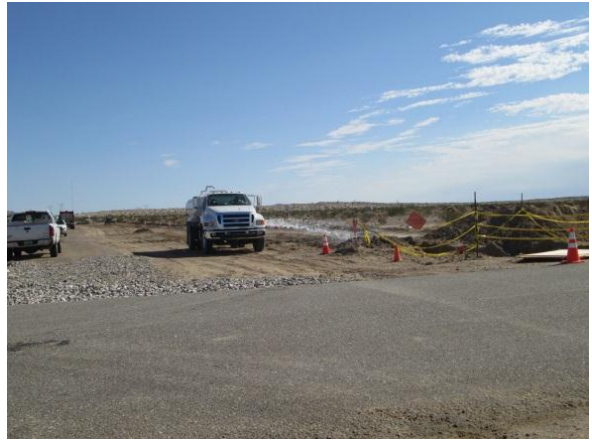
Photo 2: Stabilized construction entrances are placed at locations where project access roads intersect paved access roads in accordance with the Dust Control Plan (MM-Air-1).
