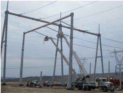
**Photo 7:** Crews complete construction of the A-Frame steel structures at the 30-acre Substation/Switchyard
