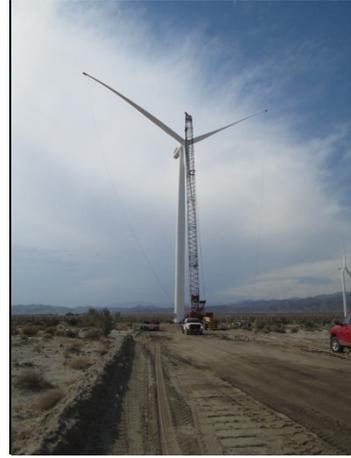
**Photo 6:** A crane is utilized to lift a rotor into place for assembly to the nacelle.
