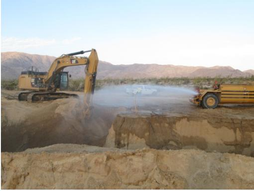
**Photo 1:** A water truck is used to suppress fugitive dust emissions during excavation activities at a wind turbine pad site in accordance with (MM-Air-1)
