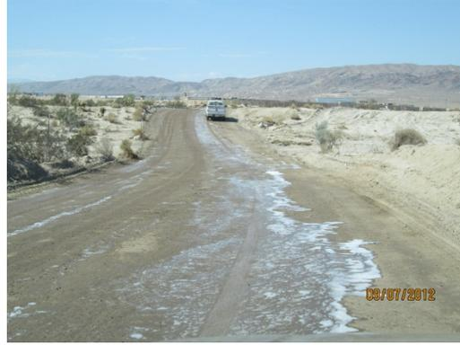
**Photo 2:** Soil stabilizers are applied to access roads to minimize fugitive dust emissions in accordance with MM-Air-1.
