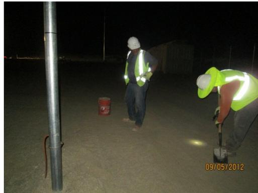
**Photo 4:** Construction crews clean a diesel leak near the 30-acre Substation/Switchyard using a spill kit in accordance with MM-Water-10.
