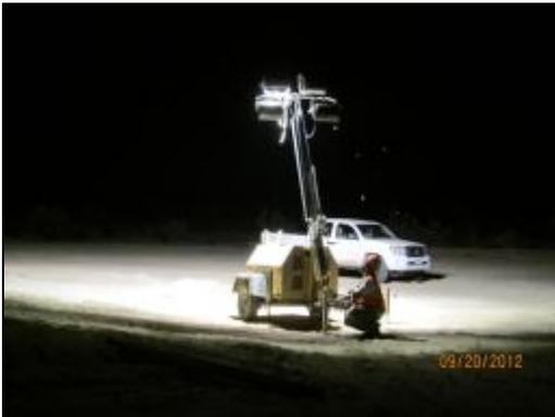
**Photo 3:** A construction worker orients lights downwards during nighttime construction activity in accordance with MM-VIS-2.
