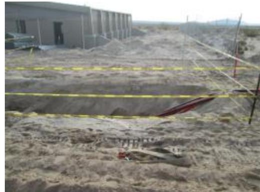
**Photo 8:** Trenching activities associated with installation of the 34.5 kV underground collection lines continue along Dos Cabezas Road adjacent to the O&M facility.
