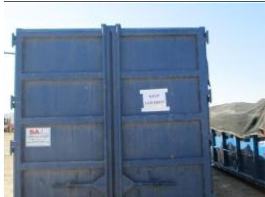
**Photo 4:** A "Keep Covered" sign is affixed to all trash receptacles to remind construction crews to securely cover trash receptacles at all times in accordance with MM-Wild-1j.
