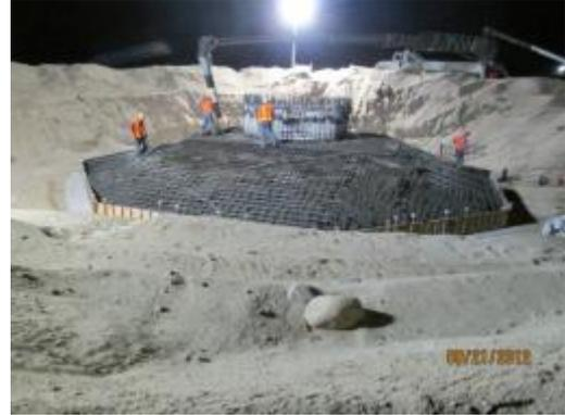
**Photo 6:** A concrete base pour is completed at a wind turbine foundation during the evening hours.
