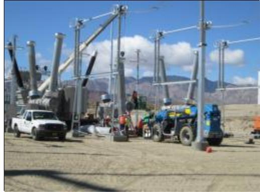
**Photo 6:** Construction crews continue installation of above-grade substation components at the 30-acre Substation/Switchyard.
