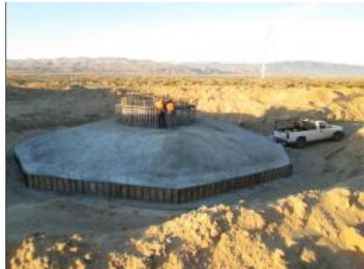
**Photo 8:** Construction crews completing construction activities at a wind turbine foundation within the approved work limits.
