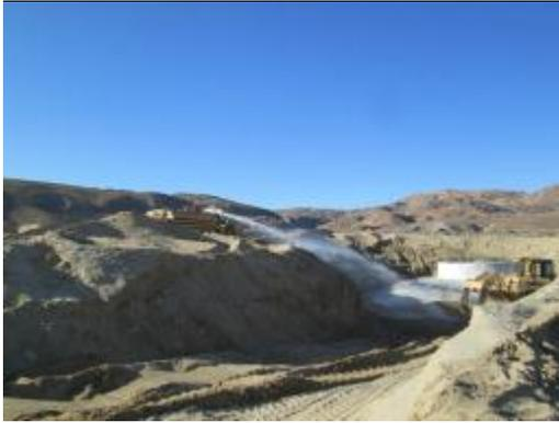
**Photo 1:** Construction crews utilize water to minimize dust emissions in accordance with the Dust Control Plan (MM-Air-1).
