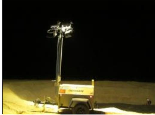
**Photo 2:** Construction lighting is oriented downward during nighttime construction work in accordance with MM VR-2.
