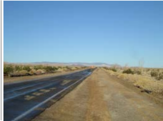
Photo 2: Trac-out is cleaned-up along County Highway S2 via use of a water truck and street sweeper.
