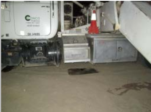
Photo 3: Drip pans are placed beneath construction equipment in accordance with MM-Haz-6 and MM-Water-9.
