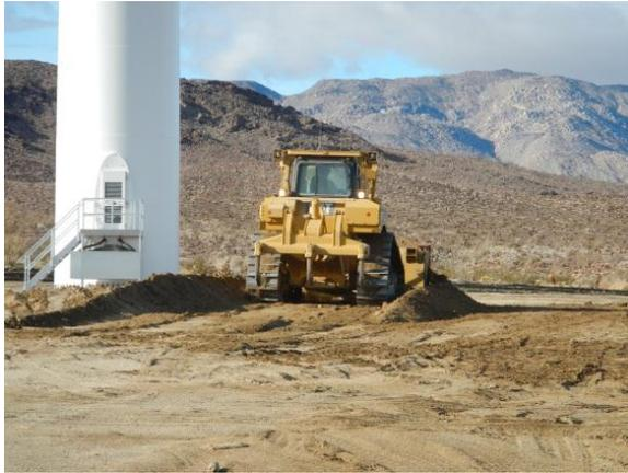
**Photo 5:** Topsoil staged onsite from initial ground disturbance is utilized to restore a wind turbine pad site in accordance with MM-Veg 2b.
