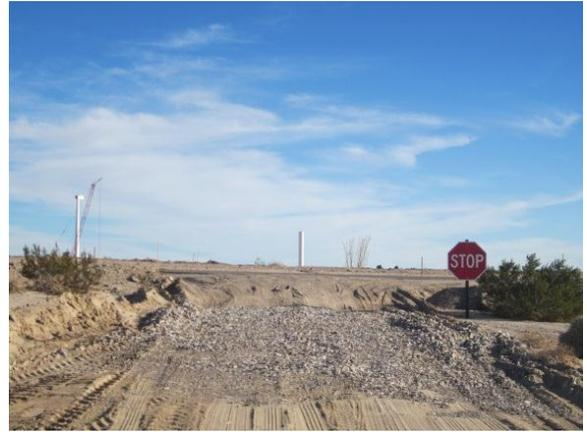
**Photo 6:** ECMs observed rock aprons being maintained to minimize trac-out along Old Mining Road in accordance with the SWPPP and MM Air-1.
