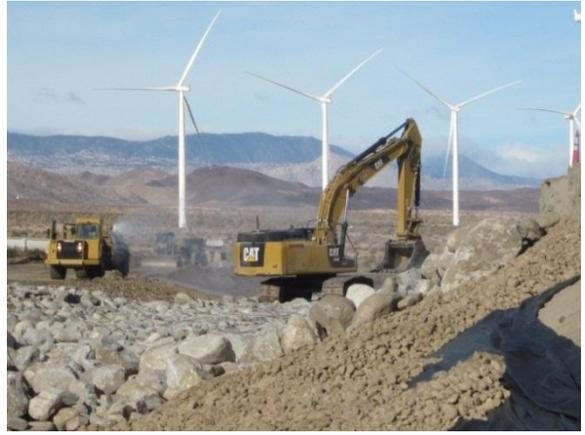
**Photo 2:** ECMS observed construction crews placing rip-rap around the substation for flood protection. Water wagons were being utilized to keep dust suppressed in accordance with MM Air-1.
