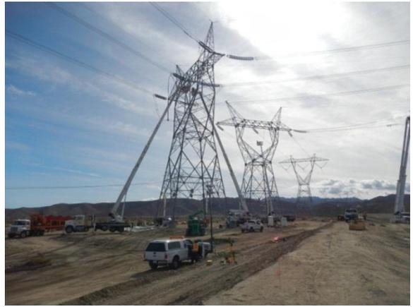
**Photo 4:** Crews were observed erecting steel lattice towers associated with the turning structures that will provide a connection from the onsite substation to the Sunrise Powerlink.
