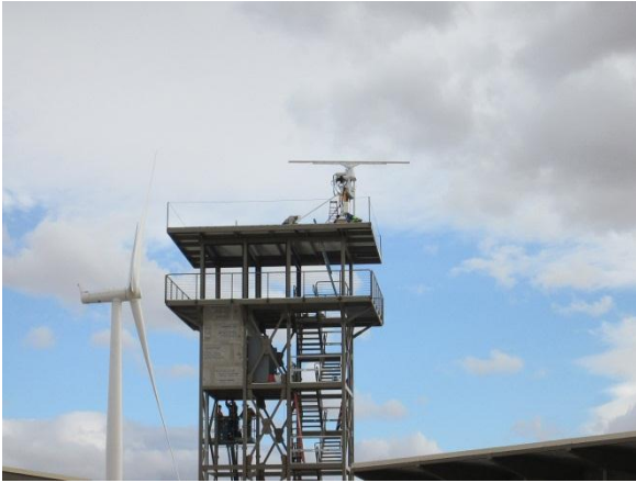
Photo 1: ECMs observed crews continuing construction activities at the ABOCC including installation of the avian radar system as identified in MM Wild-1p and the associated ABPP and ECP.
