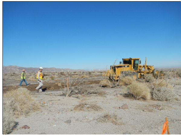
Photo 2: ECMs observed grading activities associated with the phase II substation. Both a biological and archeological monitor was present during initial ground disturbance in accordance with the ECCMP.
