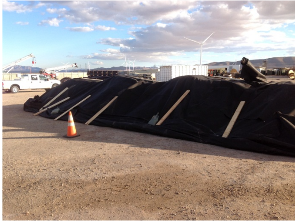
Photo 1: Soil removed from the nacelle where hydraulic fluid had been observed is contained prior to being removed offsite for proper disposal in accordance with the SPCC.
