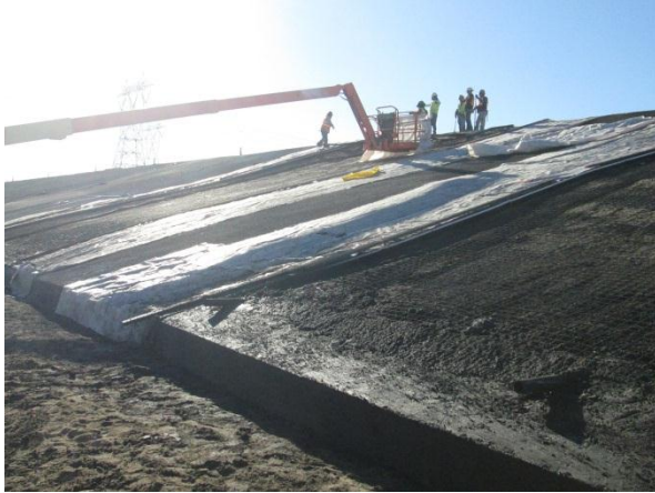
Photo 1: ECMs observe continued berm work adjacent to the SDG&E substation.
