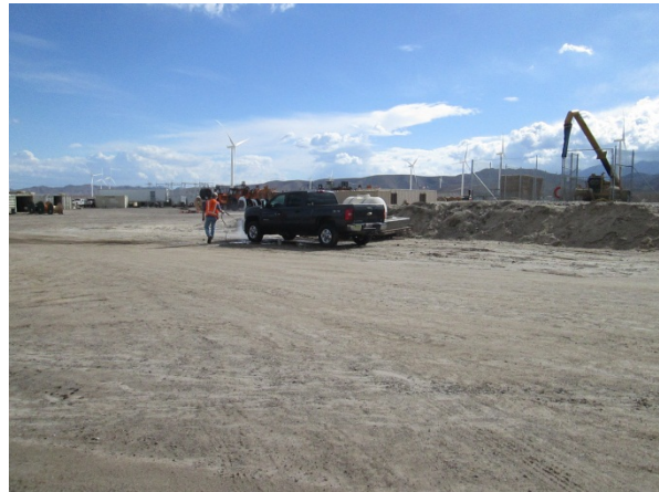
Photo 4: ECMs continued to observe wheel washing at the designated wash station in accordance with the Integrated Weed Management Plan (MM Veg-1b).
