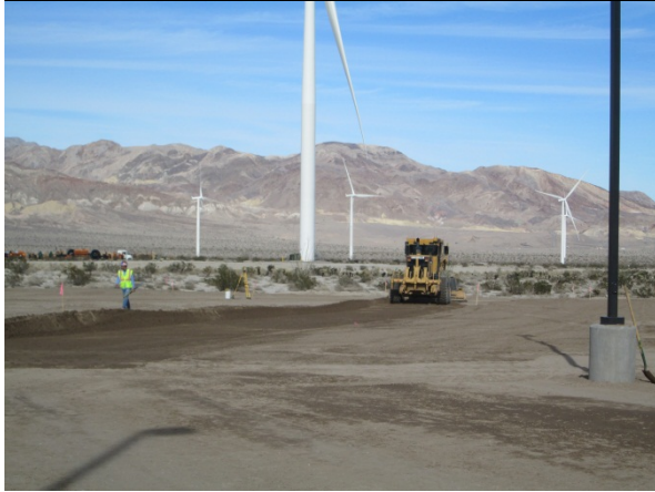
Photo 1: ECMs observed crews grading within the approved work limits at the O&M facility in preparation for paving activities. ECMs noted archaeological and biological monitors on site during initial ground disturbance.
