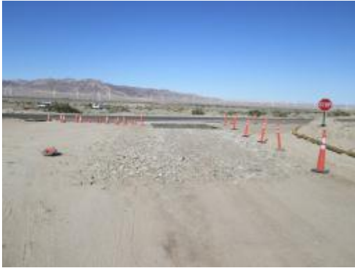
Photo 1: A stabilized construction entrance is maintained at a project entrance. The stabilized entrance consists of a rattle plate and rock apron in accordance with the Dust Control Plan (MM-Air-1) and SWPPP (MM-Water-9).
