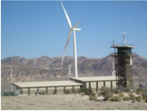
Photo 5: All exposed structural steel associated with the O&M facility is colored "Brush Brown" in accordance with the O&M Surface Treatment Plan (MM-VR-3).
