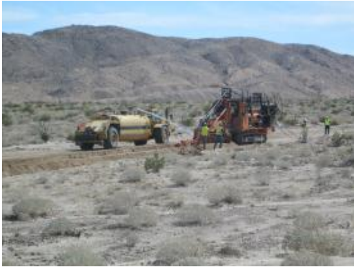
Photo 1: ECMS observed construction crews completing the installation of underground collection lines within the southern portion of the project site associated with Phase II wind turbines.
