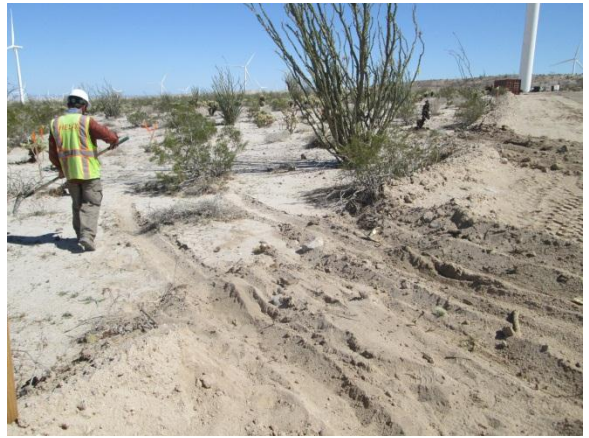
Photo 8: In accordance with MM-Veg-2b, a habitat restoration specialist restores contours associated with disturbances that occurred during tag line work as authorized by BLM in Variance 016.
