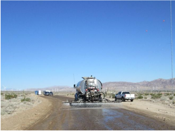
Photo 5: Water trucks were observed throughout the reporting period watering down turbine access roads in accordance with MM-Air-1.
