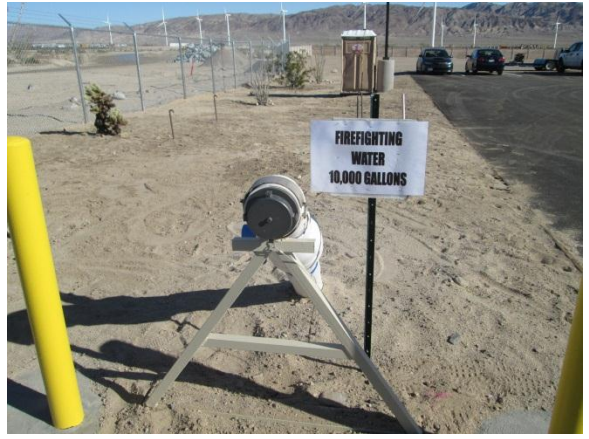
Photo 6: A source for firefighting water has been put in place at the O&M facility in accordance with MM-FF-1.
