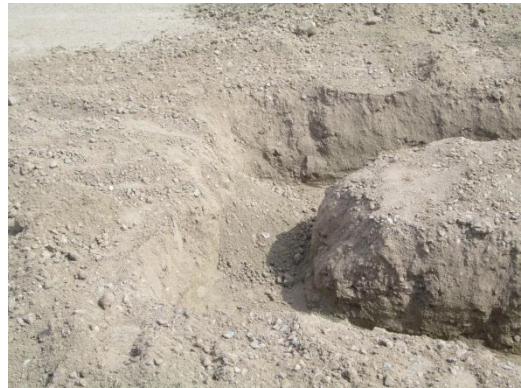
Photo 4: In accordance with MM-Wild-1b, crews place slopes at the ends of the excavations to provide wildlife escape ramps.
