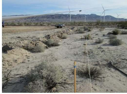
Photo 6: Stakes are utilized to delineate the approved work limits in accordance with MM-Wild-1d.
