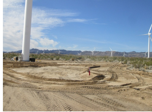
Photo 6: In accordance with MM-Veg-2b, crews place topsoil salvaged during initial ground disturbance within the limits of the temporary work areas.
