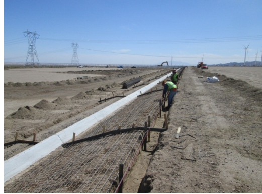
Photo 2: Construction activities associated with the berm along the perimeter of the Phase II substation continued during this reporting period.
