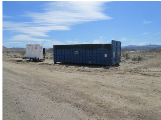
Photo 4: ECM's observed trash bins being covered in accordance with the Raven Control Plan (MM-Wild-1j) and secondary containment under portable sanitary facilities in accordance with best management practices identified in the Storm Water Pollution Prevention Plan (SWPPP) (MM-Water-9).
