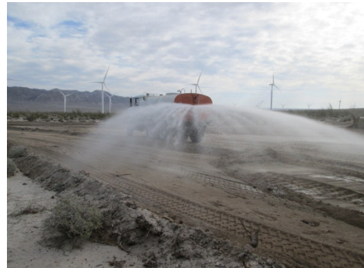
Photo 8: Water trucks are utilized to water down construction activities in accordance with MM-Air-1.
