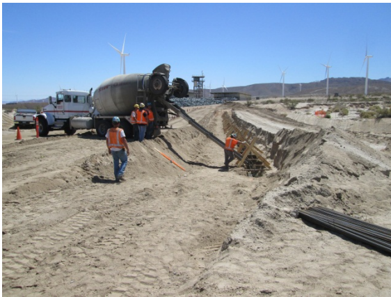
Photo 7: Construction crews construct a low water crossing on Dos Cabezas road.
