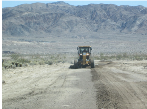
Photo 6: In accordance with MM-Veg-2b, crews place topsoil salvaged during initial ground disturbance within the temporary disturbance limits.
