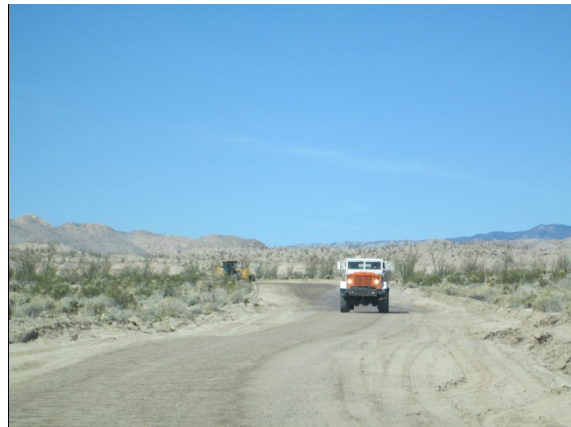
Photo 8: Water trucks are utilized to water down construction activities in accordance with MM-Air-1.
