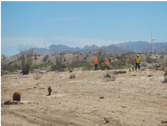
Photo 3: In accordance with Section 4.5.9 of the HRRP, vertical mulch is placed in temporary work areas to help reduce wind speed at ground level.
