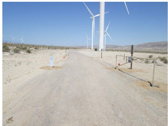
Photo 8: An access control gate and informational signage is installed to manage unauthorized access to turbine pad locations in accordance with the Access Control Plan (MM-CUL-11).
