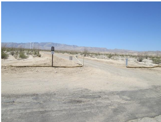
Photo 7: An access control gate and informational signage is installed to manage unauthorized motorized vehicle access to turbine pad locations in accordance with the Access Control Plan (MM-CUL-11).
