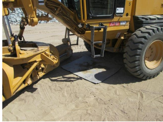
Photo 6: Drip pans are placed beneath heavy equipment in accordance with the SWPPP.
