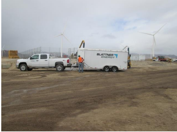
Photo 5: ECMs continued to observe wheel washing at the designated wash station in accordance with the Integrated Weed Management Plan (MM Veg-1b).
