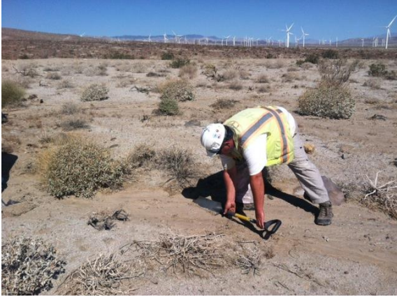
Photo 1: The lead biological monitor removes sediment discharged beyond the approved work limits to within the approved project limits.
