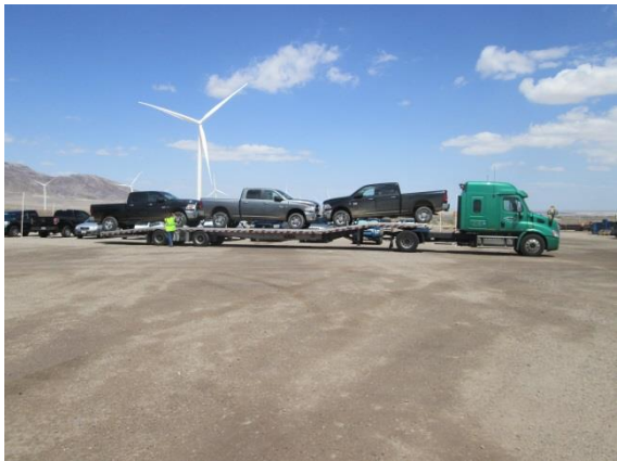
Photo 3: Construction crews continue to demobilize vehicles and equipment from the right-of-way.
