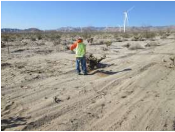
Photo 7: In accordance with Section 4.5.9 of the HRRP, vertical mulch is placed in temporary work areas to reduce wind speed at ground level.
