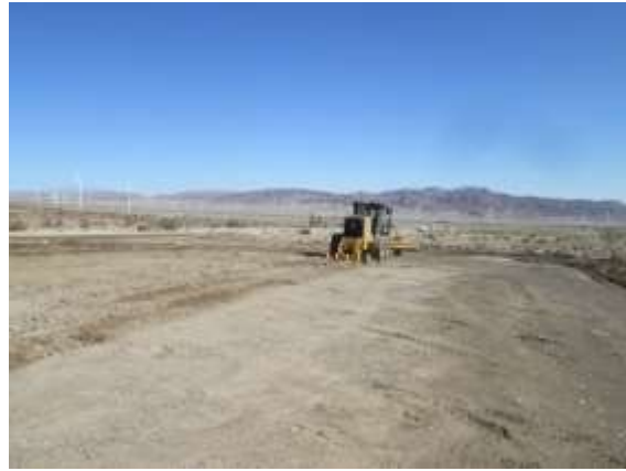
Photo 6: ECM's continued to observe reclamation activities such as soil de-compaction associated with post-construction disturbance areas within the approved work limits.
