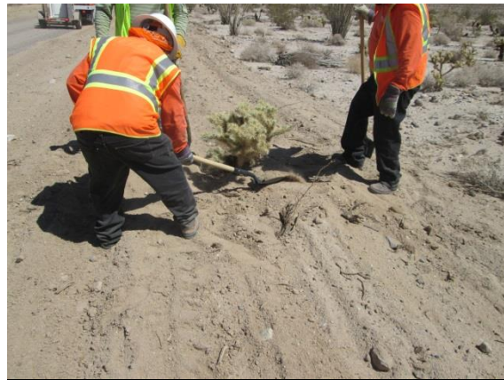
Photo 8: In accordance with Section 4.5.9 of the HRRP, vertical mulch is placed in temporary work areas to reduce wind speed at ground level.
