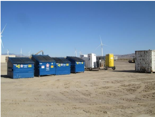
Photo 3: Trash receptacles are covered and labeled in accordance with the Raven Control Plan (MM-Wild-1j) and Construction Waste Management Plan (MM-PHS-9).
