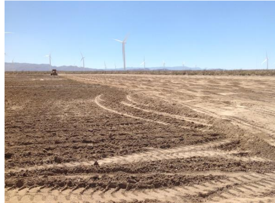
Photo 4: Construction crews complete restoration activities within the laydown yard consisting of decompacting soils in accordance with Mitigation Measure Veg-2b and the associated Habitat Restoration/Revegetation Plan (HRRP).
