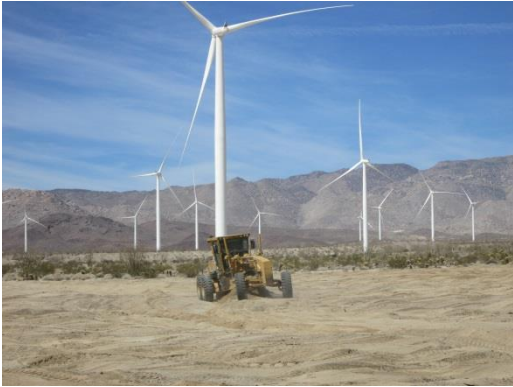
Photo 1: Construction crews completing recontouring and decompaction activities at the laydown yard in accordance with Section 4.5.2 and 4.5.3 of the Habitat Revegetation Plan (MM-Veg-2b).
