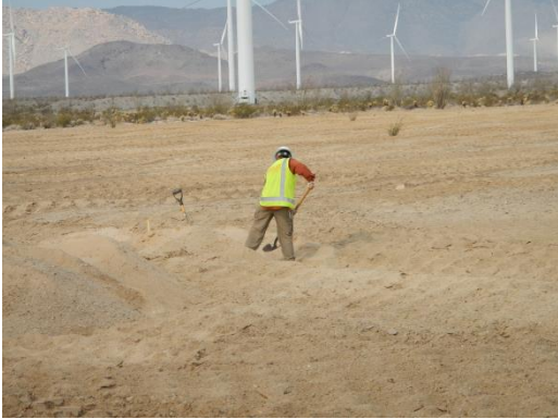
Photo 1: A revegetation specialist approved by the BLM completes recontouring of jurisdictional drainages in accordance with Section 4.5.2 of the Habitat Revegetation Plan (MM-Veg-2b).
