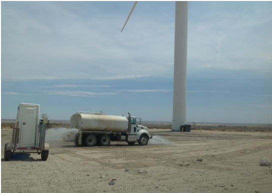
Photo 3: A water truck is utilized to pre-water a wind turbine foundation pad prior to re-disturbance activities to minimize dust emissions in accordance with the Dust Control Plan (MM-AIR-1).
