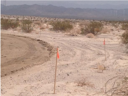
Photo 1: Staking is placed identifying the approved work limits and biological monitors are present to ensure all construction activities are completed within the approved work limits per MM-Wild-1d.
