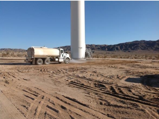
Photo 3: Water trucks are utilized during construction activities to minimize dust emissions in accordance with the Dust Control Plan (MM-AIR-1).
