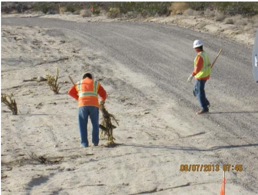
Photo 7: In accordance with Section 4.5.9 of the HRRP vertical mulch is placed in temporary work areas to reduce wind speed at ground level (MM-VEG-2B).
