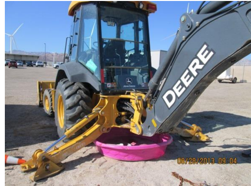
Photo 4: Secondary containment was placed under construction equipment staged along the right-of-way to minimize the potential for equipment fluids to be discharged onto the ground in accordance with the SWPPP (MM-HYD-9).
