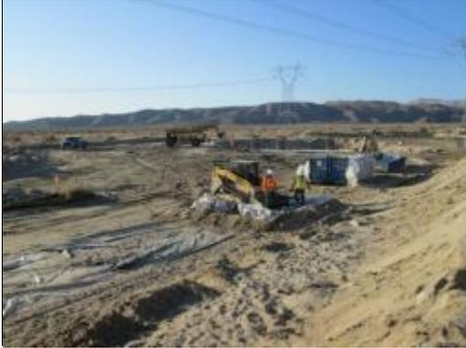
**Photo 5:** The secondary containment from a concrete washout basin is properly disposed of in accordance with the Construction Waste Management Plan (MM-PHS-9).
