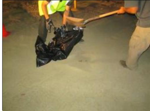
**Photo 2:** An oil leak is properly cleaned-up and disposed of in accordance with the SWPPP (MM-Water-9) during the evening hours.
