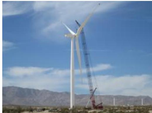
**Photo 8:** A large crane is utilized to lift a rotor into place.
