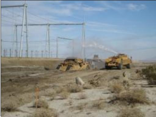
**Photo 1:** Construction crews utilize water to minimize dust emissions during grading activities at the 30-acre Substation/Switchyard in accordance with the Dust Control Plan (MM-Air-1).
