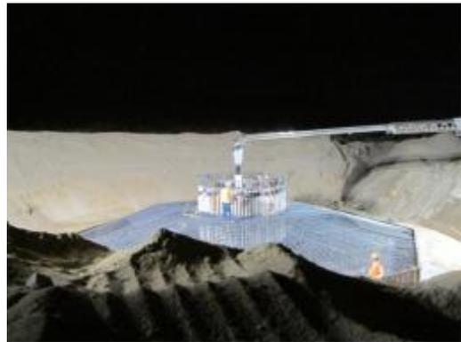
**Photo 4:** A concrete base pour is completed at a wind turbine foundation during the evening hours.
