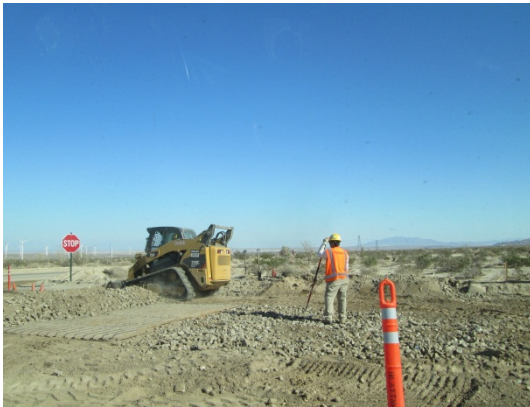
Photo 3: Workers repair the stabilized entrance to Dos Cabezas Road.
