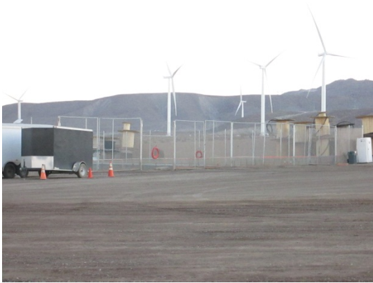
Photo 7: Gates to the temporary water pond are closed during periods of minimal activity at the laydown yard.
