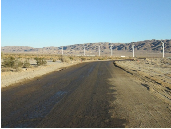
Photo 5: Dos Cabezas road is watered to keep dust suppressed in accordance with the Dust Control Plan (Mitigation Measure Air-1).
