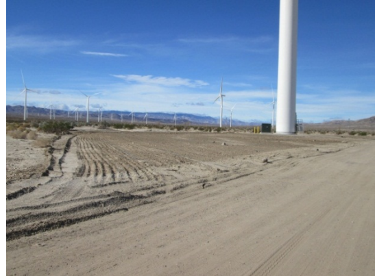
Photo 8: Previously disturbed top soil is used to restore a wind turbine pad site in accordance with Mitigation Measure Veg-2b and the associated Habitat Restoration/Re-vegetation Plan.
