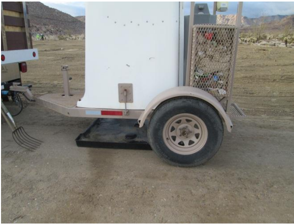
Photo 3: Secondary containment is placed beneath portable toilets onsite to prevent soil contamination per the SWPPP and Mitigation Measure Water-10.
