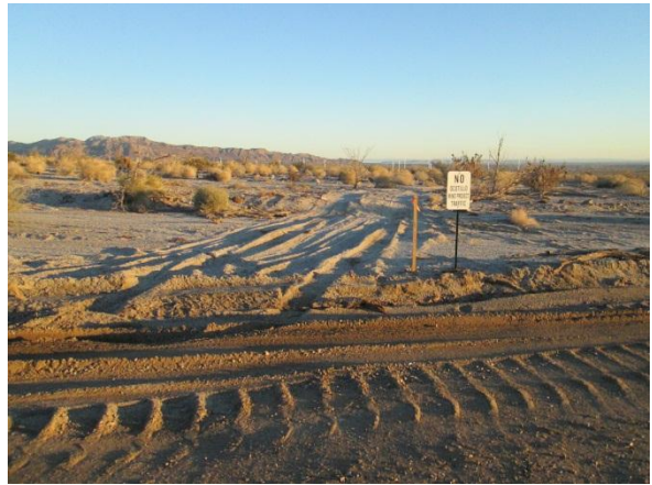
Photo 4: No access signs for non-project approved roads are placed onsite to notify construction workers that no access is permitted beyond the approved work limits.
