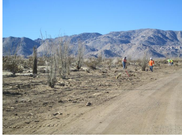
Photo 2: ECMs observed crews utilizing vertical mulching techniques to restore disturbed areas in accordance with the Habitat Re-vegetation plan (MM Veg-2b).
