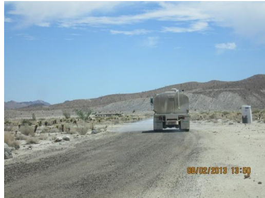
Photo 4: Water trucks are being utilized along access roads to minimize dust emissions in accordance with the Dust Control Plan (MM-AIR-1).
