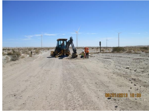
Photo 2: Crews reinforce access control gates located at the entrances to wind turbine pad sites. The access control gates are required in accordance with the Access Control Plan approved by the BLM (MM-CUL-11).
